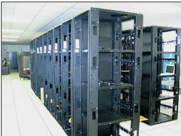
Fig. 8 - The rack-mount housing
